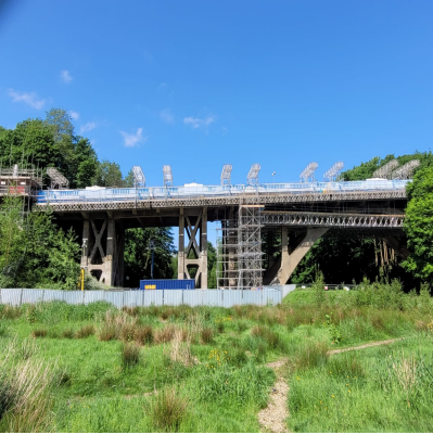
Queens Park Road Bridge
