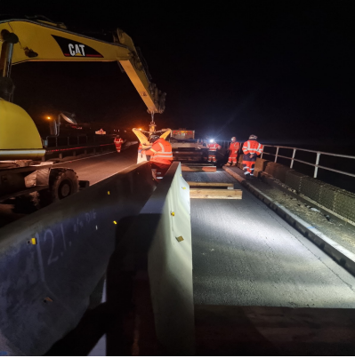
Salters Brook Bridge
